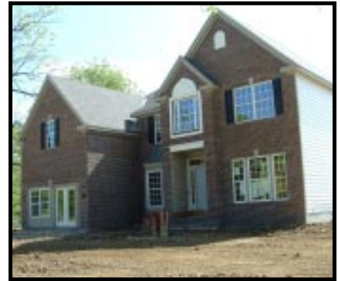
The model home at the Estates at Blackhawk is nearing completion.
