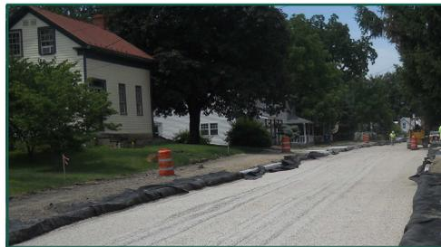
road will not be usable for a week while the concrete cures. Brick is being delivered and setting will begin soon. *Work is progressing on rebuilding Walnut St. with pervious pavers.*
